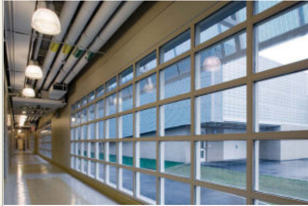
Facility spaces are aligned along a common glass-walled corridor, which encloses the facility's internal courtyard.
